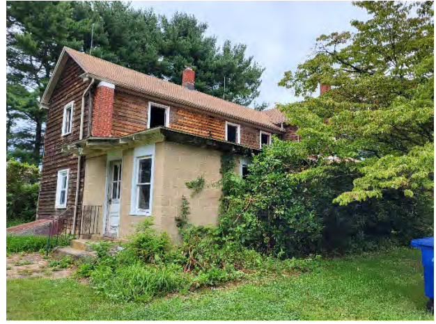
Existing House (Back).
